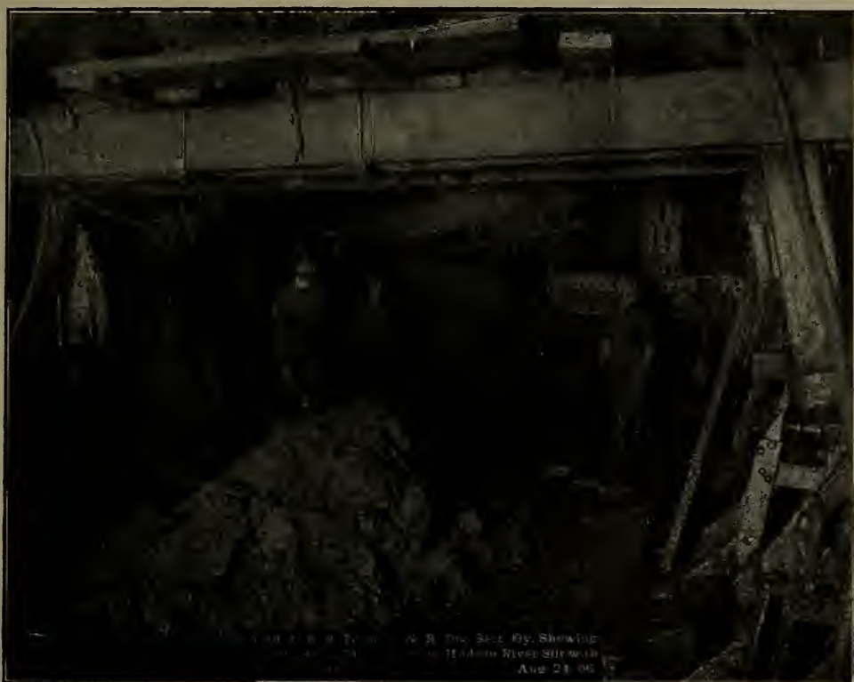
Interior of Shield in P.R.R. North River Tunnel, Showing Silt Entering Through One Open Door.
